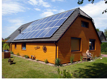
Off grid power system
